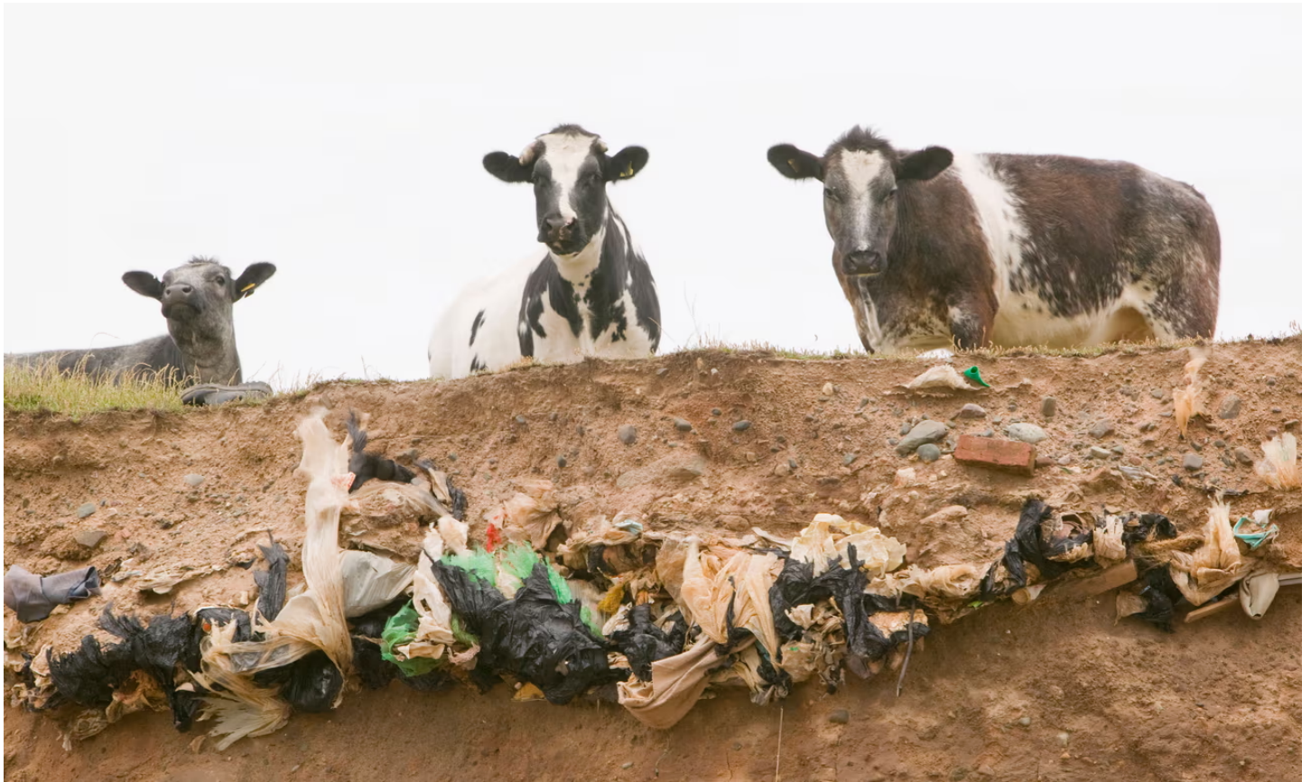
Old landfill rubbish is revealed by coastal erosion of a sea cliff on Walney Island, Cumbria, UK.
